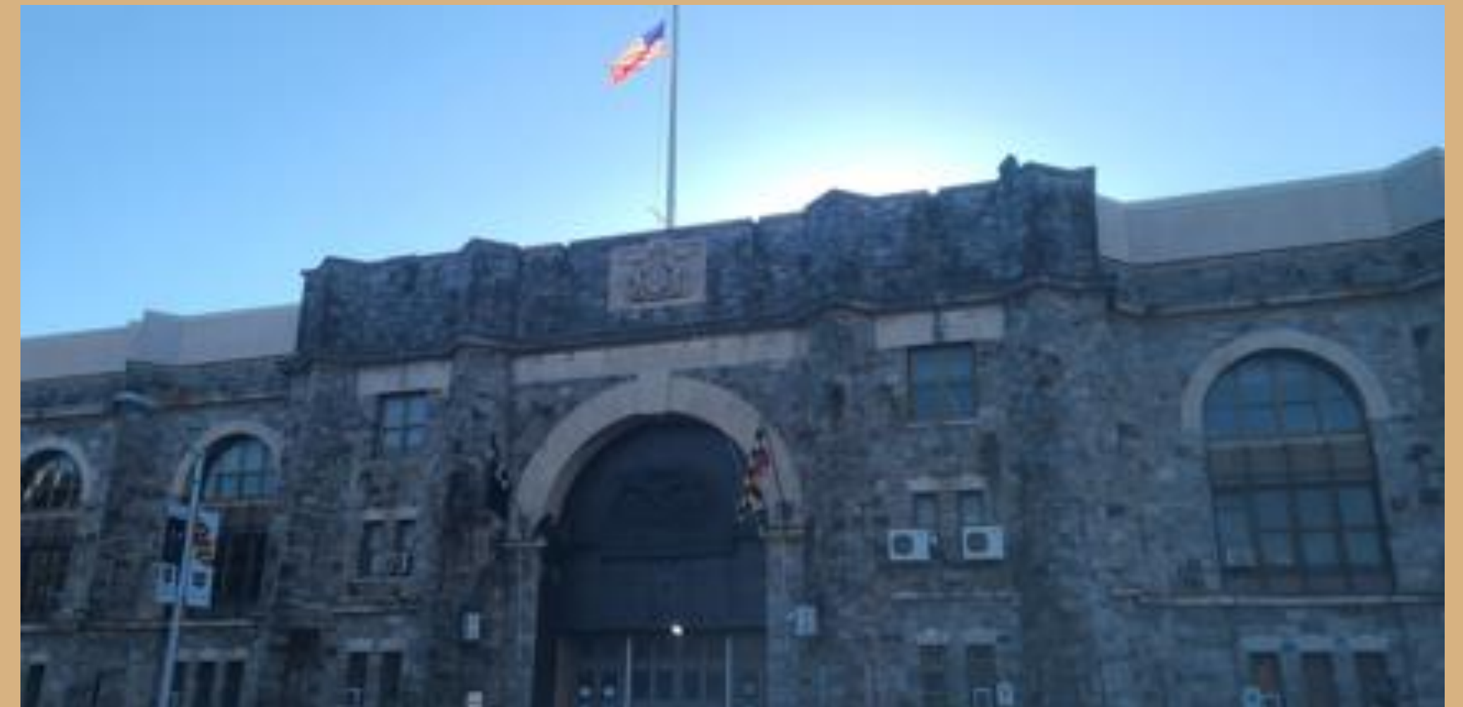
Picture of Fifth Regiment Armory (site building) taken on day of inspection (above).
